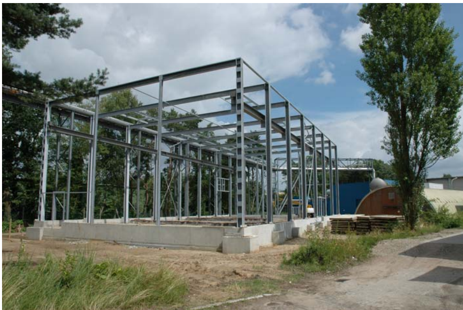
Fig.1: CMTB-experimental hall, status 23 July, 2005
