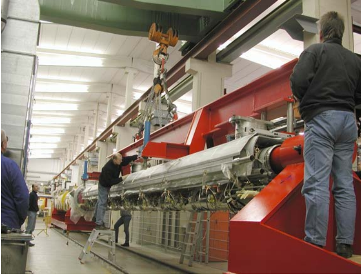
Fig. A.5.6 : Cold-mass and cavity-string in cantilever
