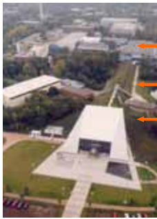
TESLA Test Facility (TTF 1, 1995-2002) TTF 2 experimental hall
